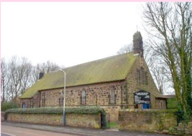
St. John's Backworth
