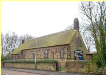
St. John's Backworth
