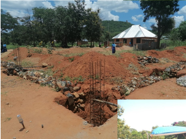
The foundations of the new church
