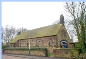
St. John's Backworth
