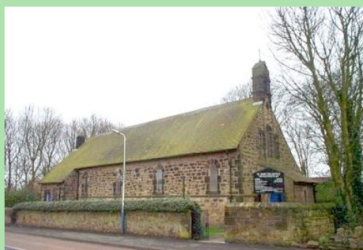
St. John's Backworth
