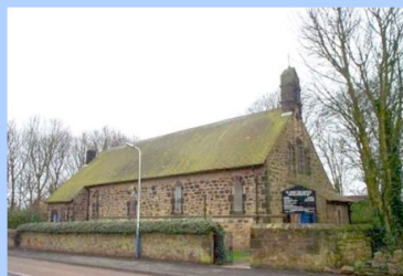
St. John's Backworth
