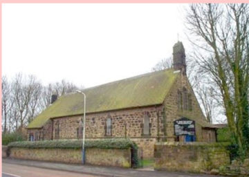
St. John's Backworth
